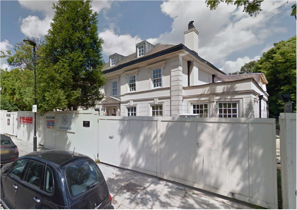
Subject building as seen from Woronzow Road
