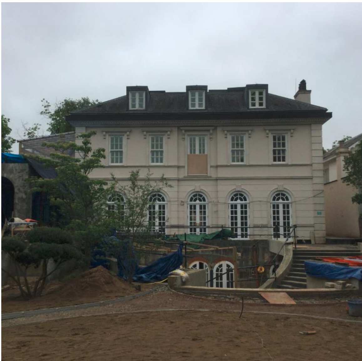
Rear of subject building.
